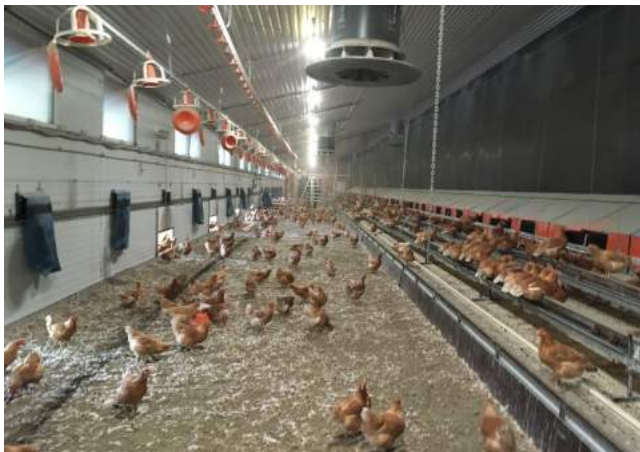
House with Pollux lighting system (left side)
